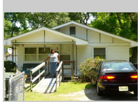
Workforce housing targets families who earn between 80 and 120 percent of the area's median income.
