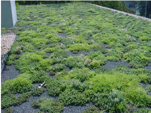
Figure NR2: Furman Office Building, Greenville SC.
