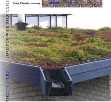
top: Tree box filters – Source: Stormtree middle: Green Roof – Source: Wikimedia Commons bottom: Permeable pavement - private parking and public right-of-way applications
