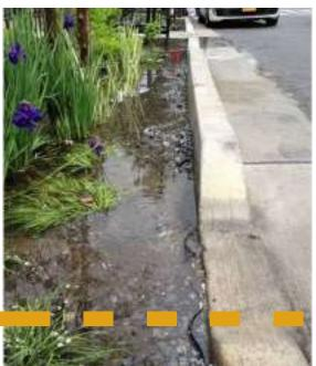
right. Bioretention within the right-of-way
